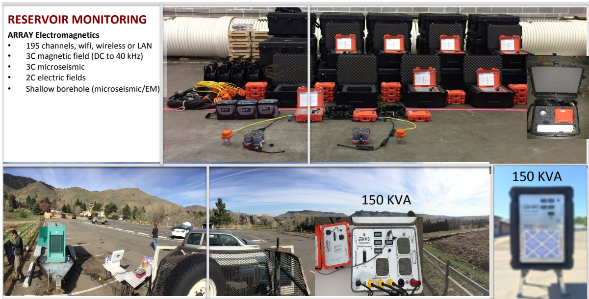
Figure 6 The electromagnetic acquisition system for monitoring example showing transmitter and the 195 channel receivers.
